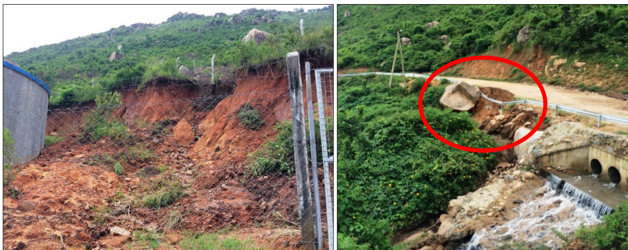
Figure 50: The effects increased flows had on the water quality and infrastructure. Large material such as boulders may cause damage to the infrastructure as seen in the above image (circled in red).
