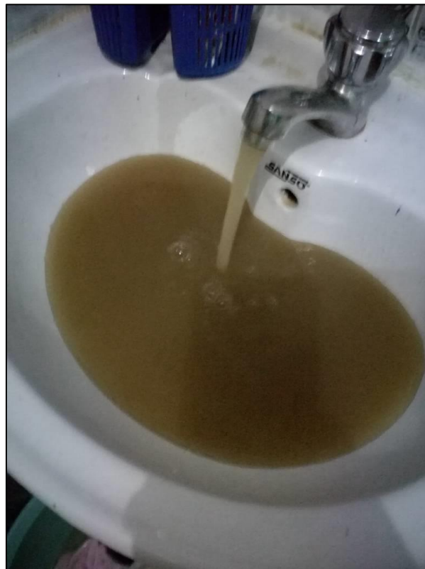
Figure 22: The effects increased flows had on drinking water quality (Photo courtesy: MWAUWASA water utility).
