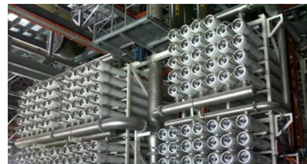
One of the reverse osmosis trains at Singapore's NEWater Plant Source: http://www.biwater.com
